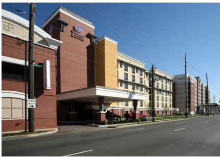
ABOVE: The Comfort Suites City Centre is about 500 feet from the entrance to the Lucas Oil Stadium, site of the Final Four.
